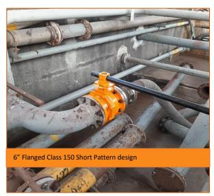
**SNR technologies** received a requirement from a chemical company to provide a solution for an old 6" Class 150 short pattern ball valve. The requirement was generated after an incident where the process valve heavily leaked in-line. Due to a lack of support from the valve manufacturer, and no spare parts available for maintenance, it was decided to replace the valve with a new product.
